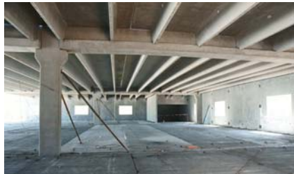
View across four classrooms - ready for other trades to begin work
