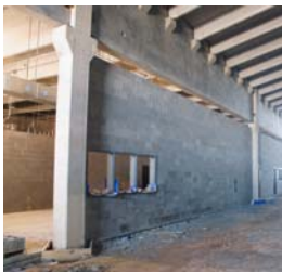
Column/beam line with CMU demising wall
