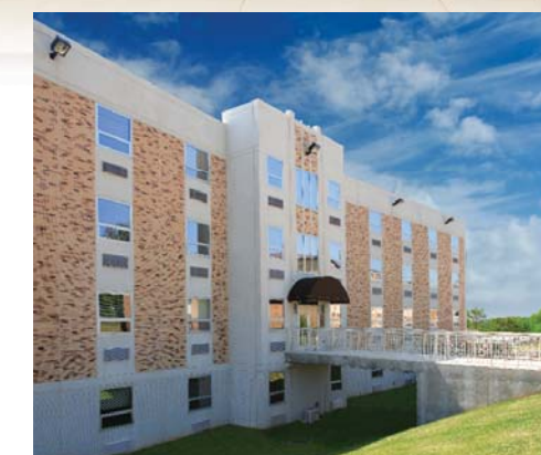
Four level, total precast student dormitory with a capacity of 120 beds
