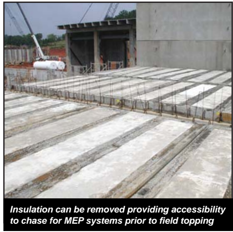
Thin floor plate is ideal for platform or podium construction in mixed-use projects
