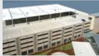
Integrated Rainwater Collection
